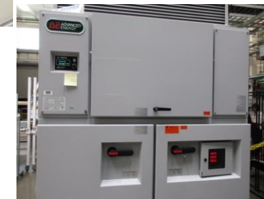
Comparable AE inverter to those installed at PMRF
