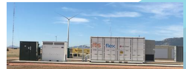
430 kW PV array Scaled to 19.3 MW
