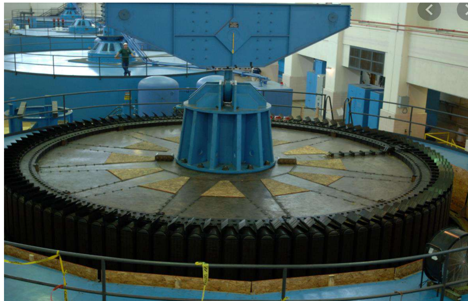
Extreme Large Rotating Mass of a Kaplan Turbine/Generator Unit
