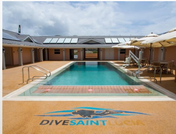
Harbor Club Dive School LEED BC+D V3
