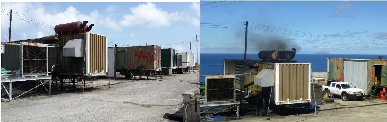
*Picture 8: Current Generators Utilized for Electricity Production at Montserrat Utilities Limited.<sup>19</sup>*
