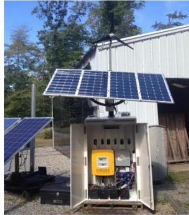
The Joule Box is a portable power unit which provides solar, wind, battery & hydrogen power. Can be plugged into an 110v outlet, can be configured to any size.
